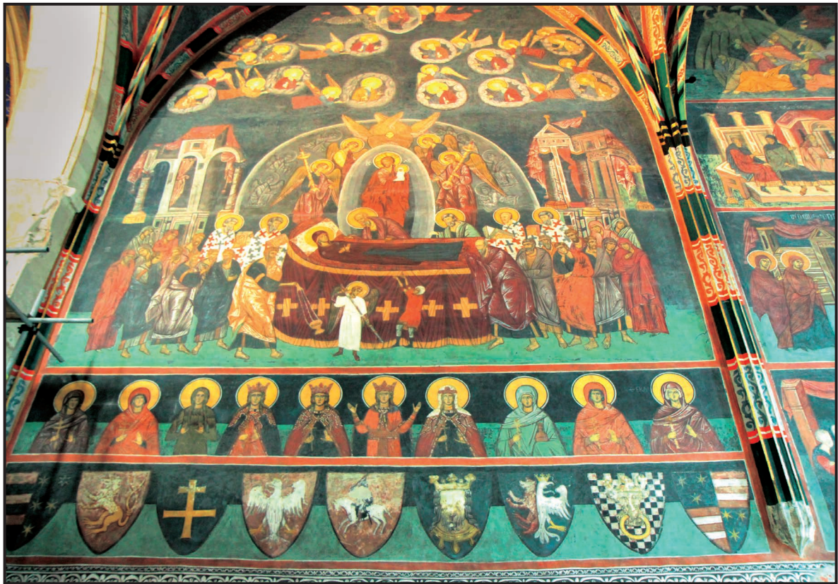
Fig. I. Northern wall of the presbytery upon conservation. A photo by Rev. Andrzej Rusak
